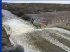
Rye Patch Dam Photo April 2017 - Courtesy NDWR Dam Safety
