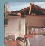
House destroyed by channel migration on the Carson River in Lyon County, Nevada 1997
